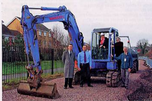
Morrisons, here we come! From left: Andrew Dakin (Pride in Barry), John Buxton (project manager), Jane Hutt (Welsh Assembly), Margaret Alexander (Vale of Glamorgan Council) and Brian Mills (Barry Island Heritage Railway), inspect work on the 500-metre extension. MARK LANG
